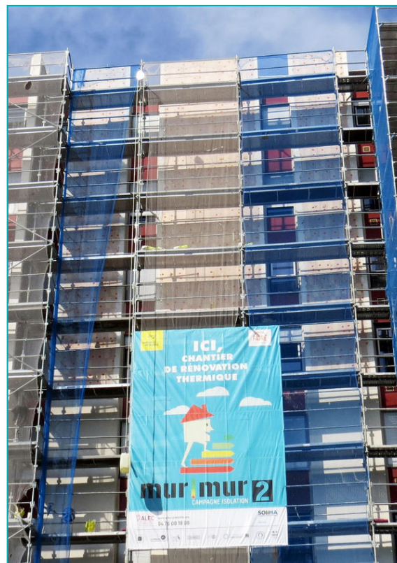
Building being retrofitted under Mur | Mur (© Grenoble-Alpes Métropole)
